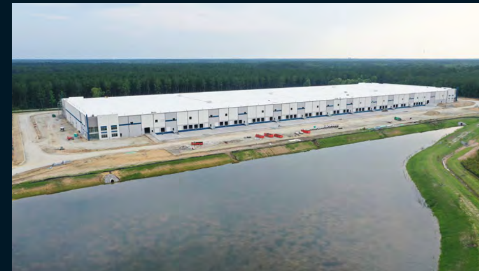
Concrete Truck Court and Drive Aisle
