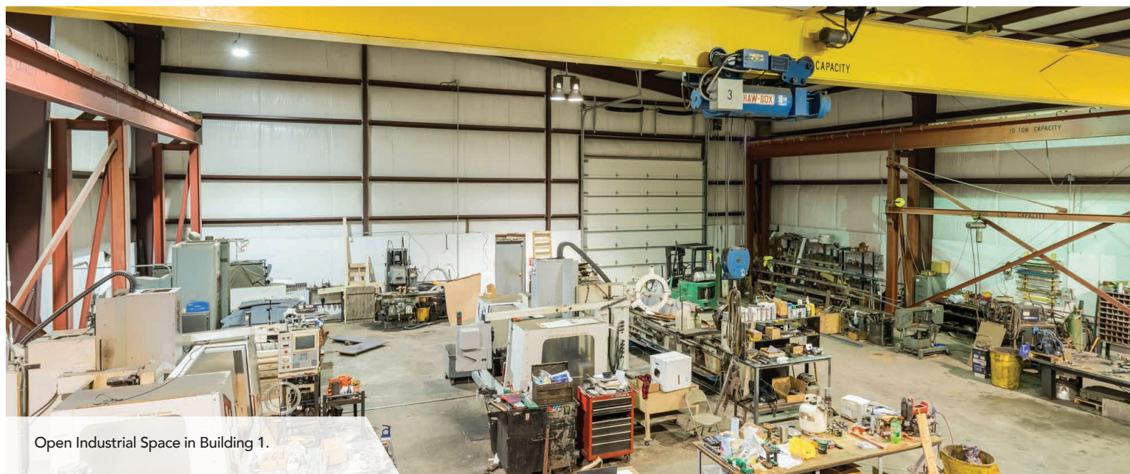
Industrial Space in Building 1.
