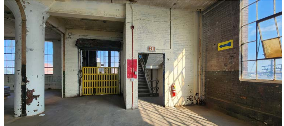
FREIGHT ELEVATOR & MAIN STAIRWELL ACCESS
