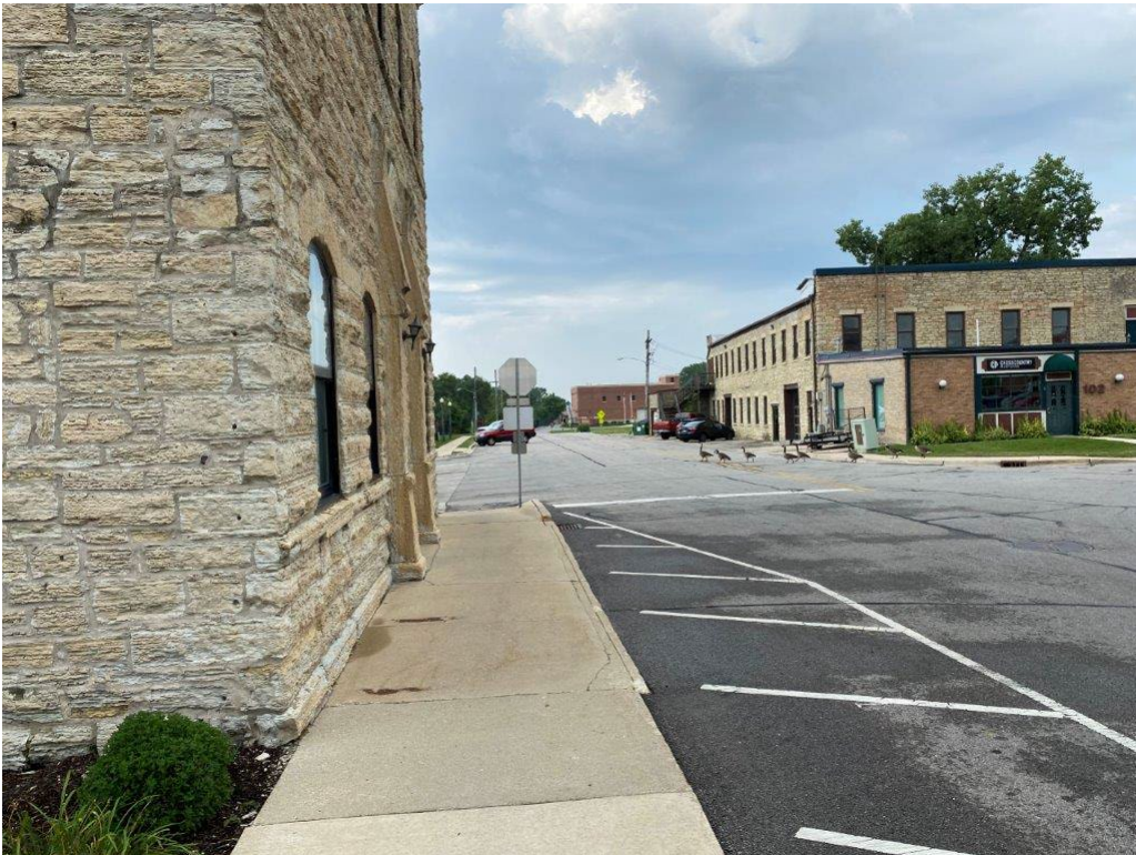
Street Scene - Facing Southerly Along South Shumway Avenue
