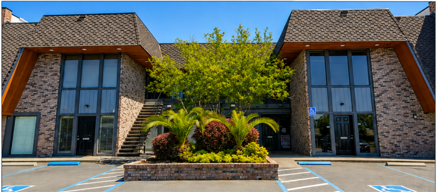
Main Office Building
