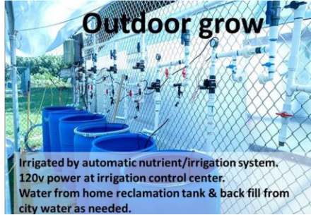
Automatic nutrient/irrigation system, with water reclamation
