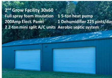
2nd Grow Facility 30x60 200Amp 2 2ton mini split 1 5ton heat pump
