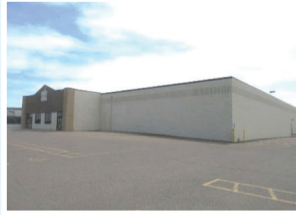
FRONT FACING SOUTHEAST
