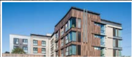
PARK JAMES HOTEL 60 ROOMS | OPENED 2018
