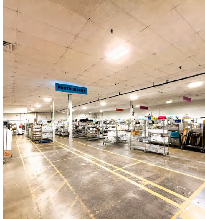
Middle Bay with Drop Ceiling
