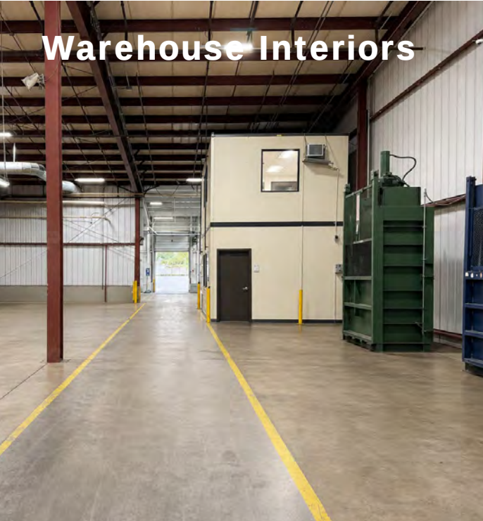
South Bay Facing Loading Docks
