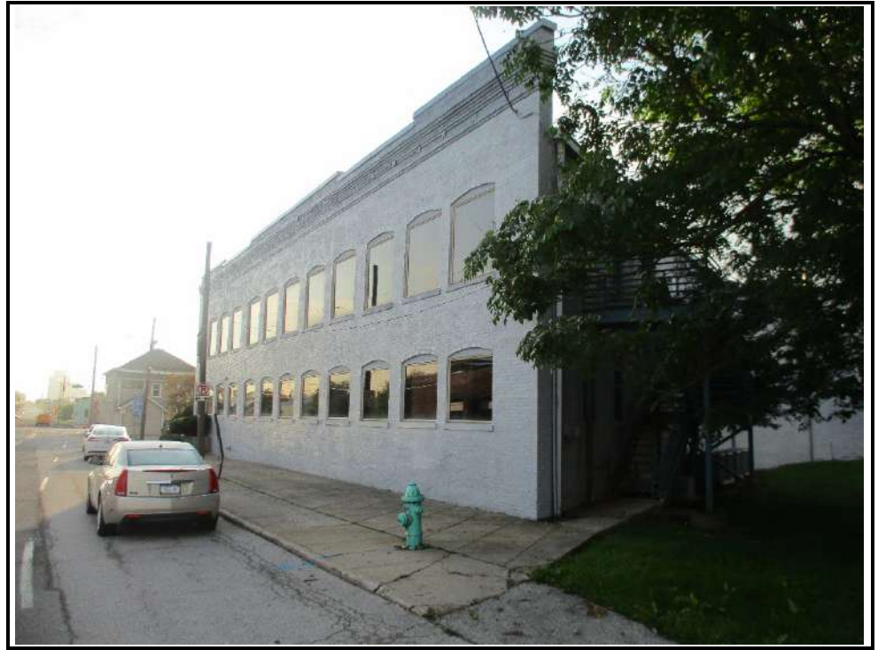
North (Front) and West Elevations From McCarty Street
