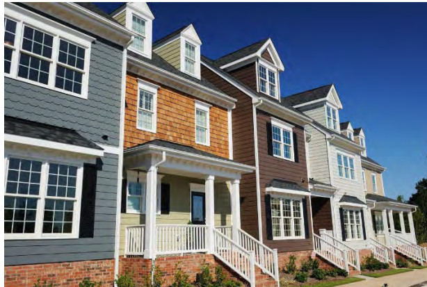
These units have a slab foundation that is raised at least 18 inches and is clad in brick.
