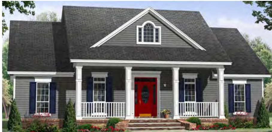
This house has a slab foundation that is raised an average of 18 inches from the ground, and the foundation is clad with brick.
