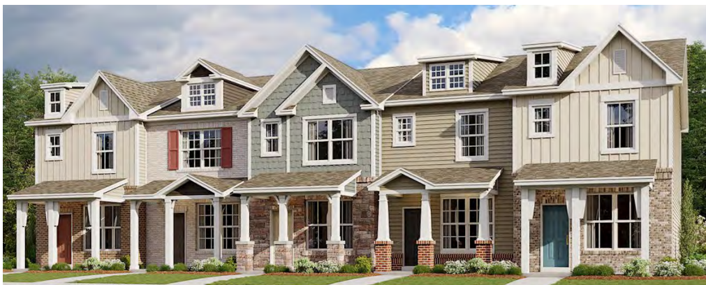
These units have a slab-on-grade foundation but each unit is clad with at least 18 inches of brick from the ground.
