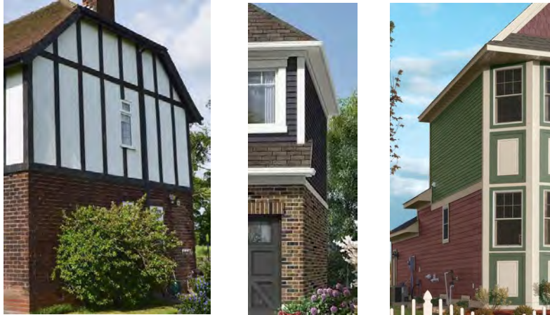
These homes have a band of contrasting color between the stories and at the corners, and the upper story is different from the lower story in terms of materials or color.
