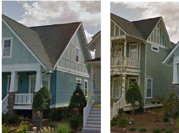
These three homes have a band of contrasting color at the bottom of the gable area, and the area within the gable contains siding of different material or shape.
