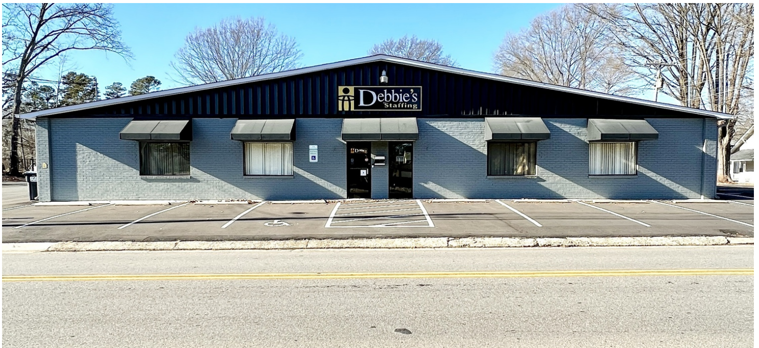
Suite A - Front view of building
