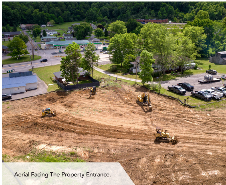
Aerial Facing North.
