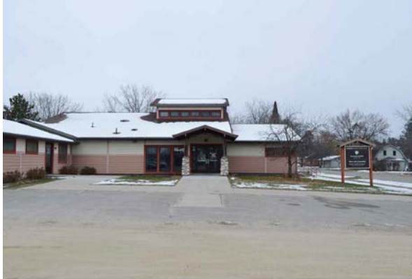
Front/South Side of Bldg - Main Entrance
