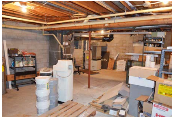
Lower Level - Utility
