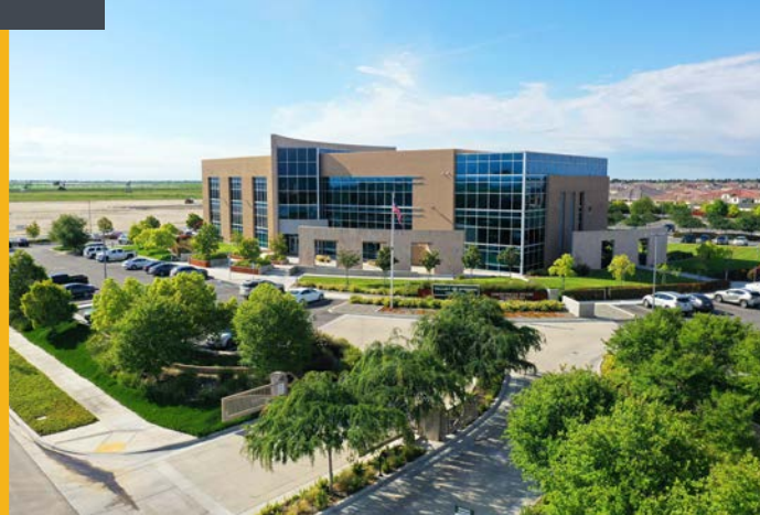
Valley Strong Credit Union 60,000 SF Headquarters
