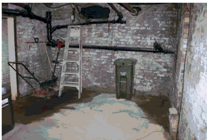
Basement Storage / Water leak
