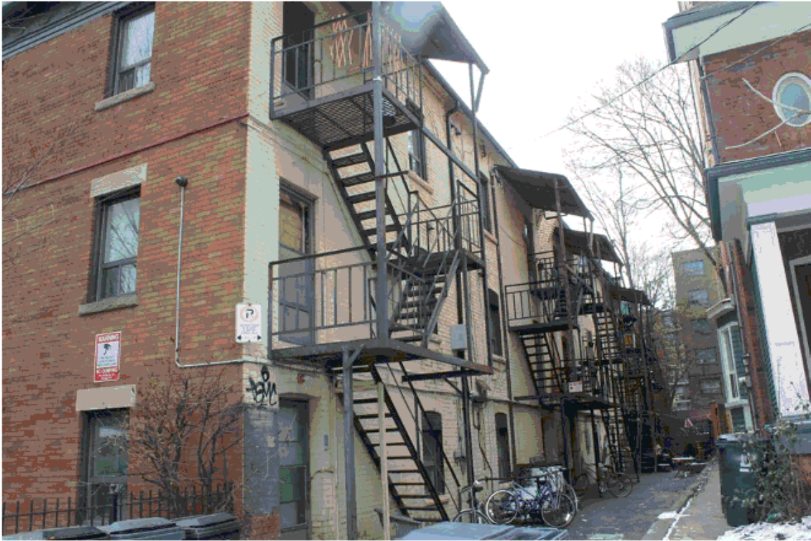
1384-1386 KING STREET WEST – REAR (NORTH) ELEVATION
