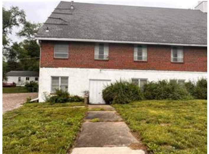
south basement entrance
