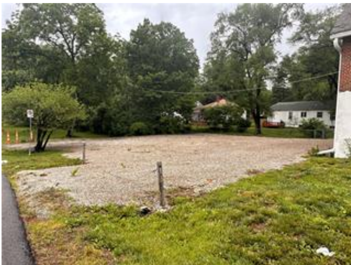
overflow parking lot
