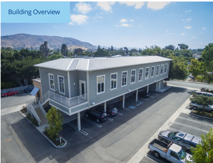
Pismo Street Frontage
