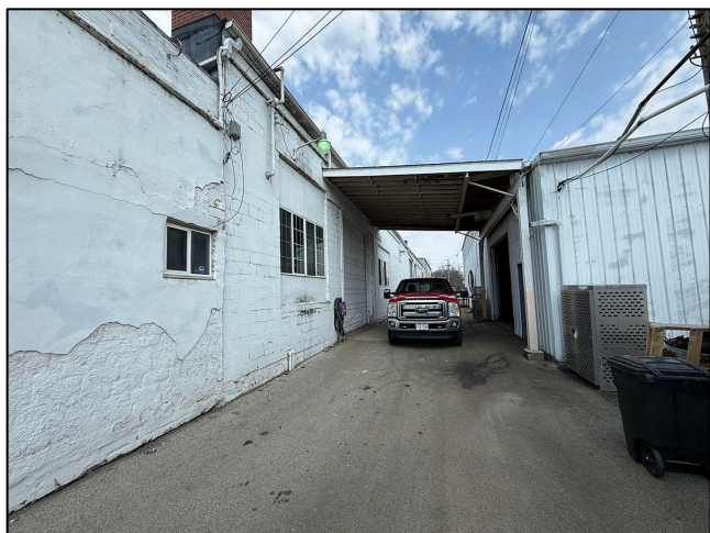
Delivery access through alley. Overhead door (13'7" x 14")
