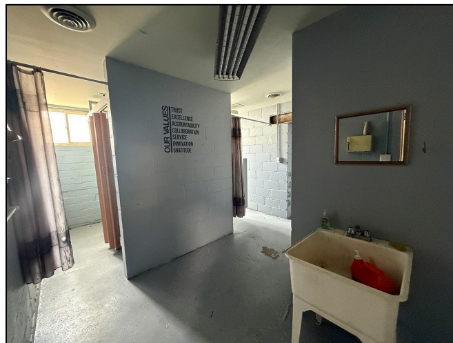
Men's locker room
