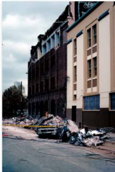
Earthquake shaking caused the unreinforced brick parapet and façade of this building to collapse, killing people on the ground.
