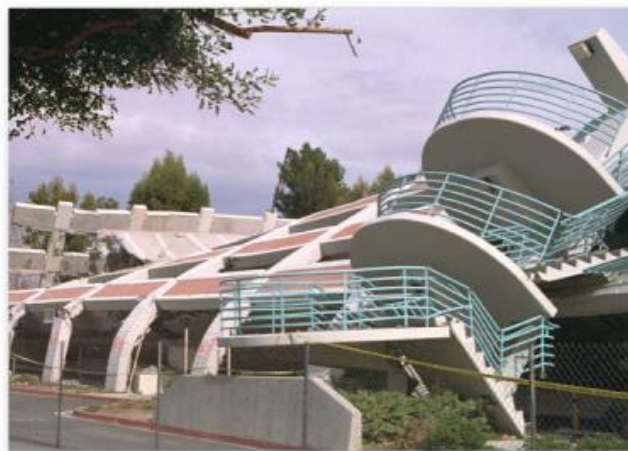
Concrete columns with inadequate confining reinforcement steel failed during the 1994 Northridge earthquake.
