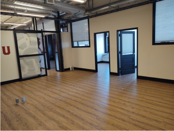
South work area
