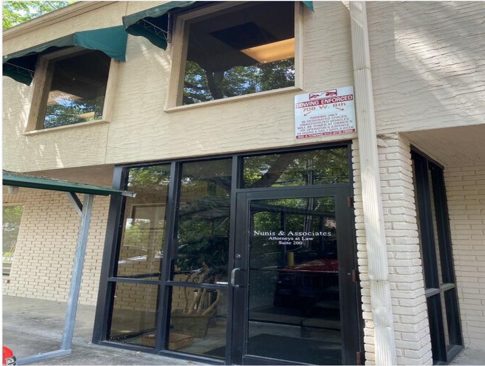
Front of building to office space.
