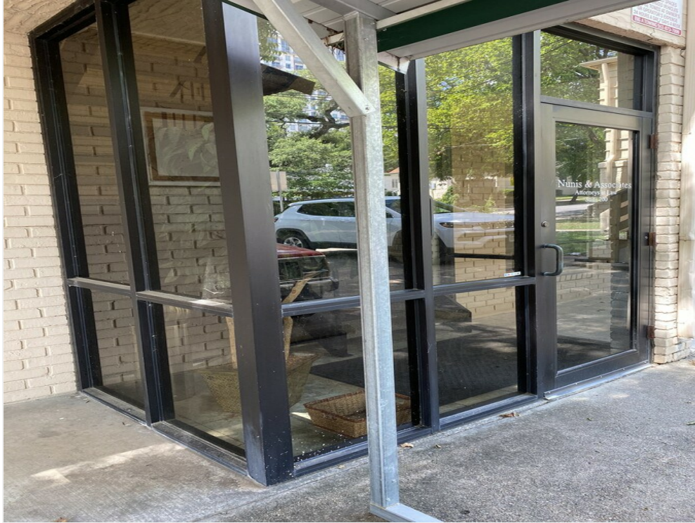
Front of building to office space.
