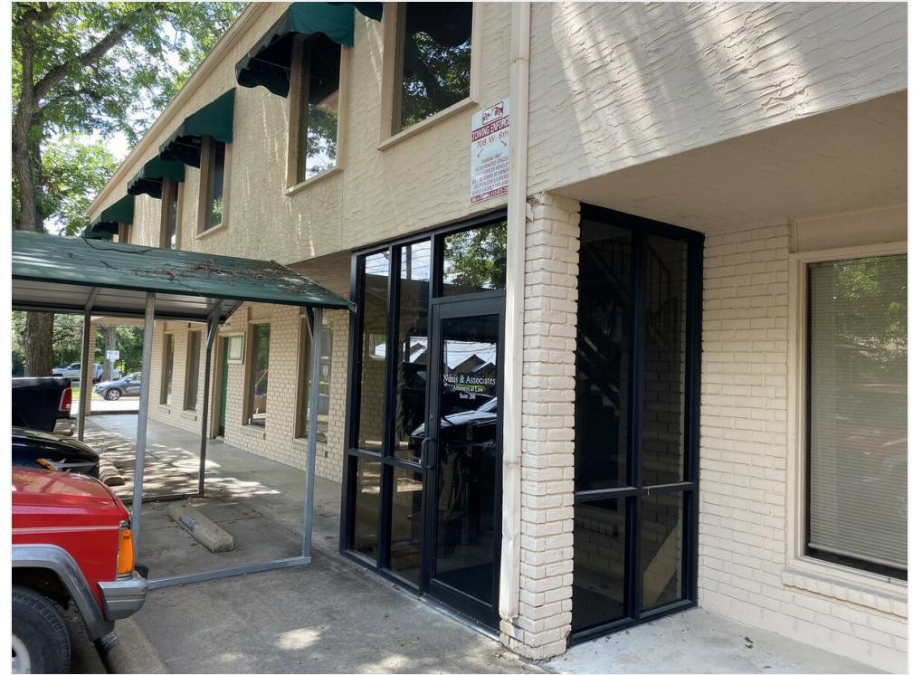
Front of building to office space.
