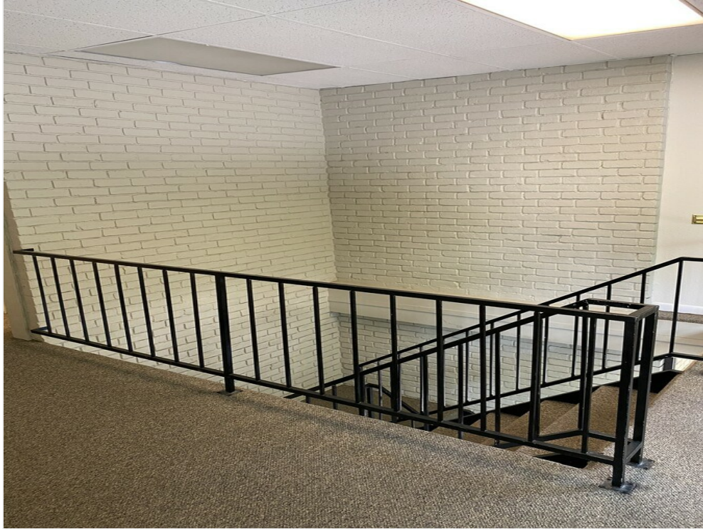
Top of stairwell.
