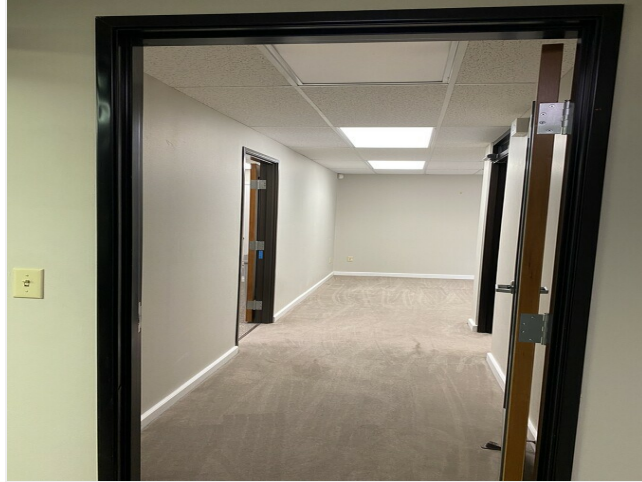
Door to close back offices from front office, kitchen and lobby.
