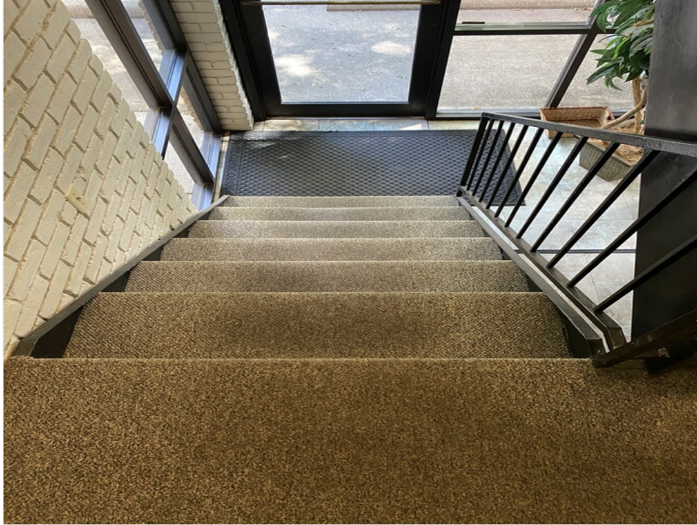
Stairwell facing entry.
