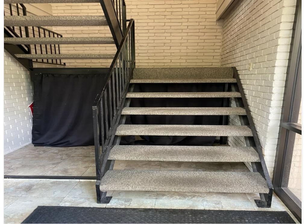
Stairwell to office space.
