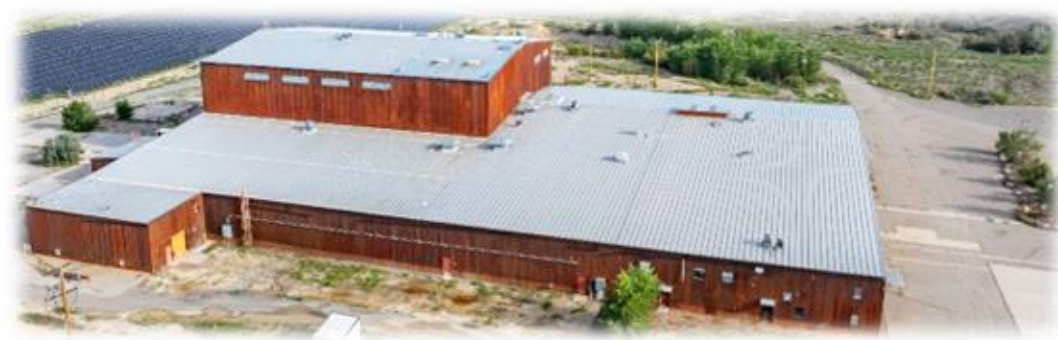
View of Facility facing South
