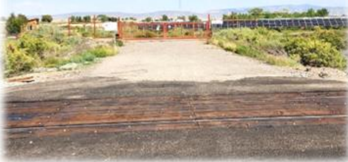
Automated Security Gate/RR Tracks
