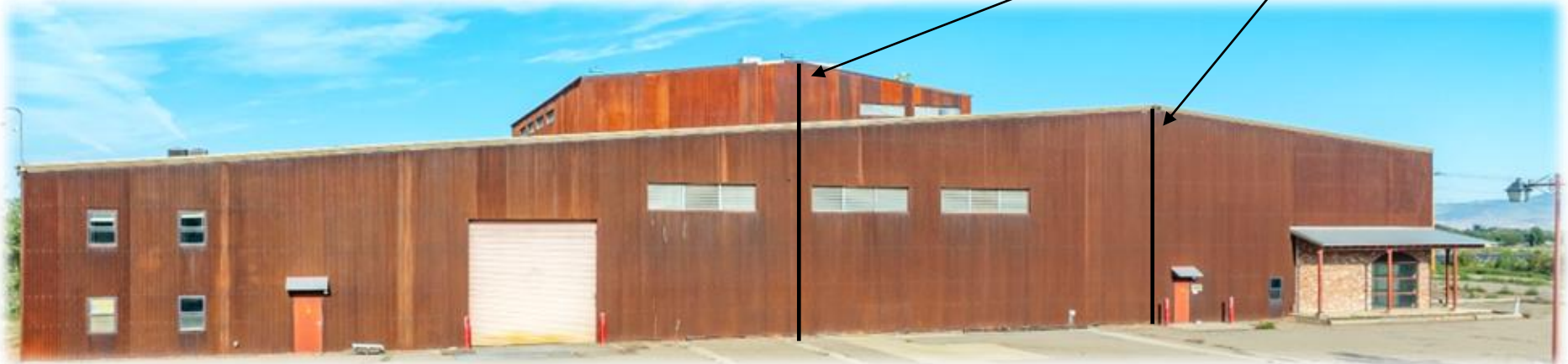
View of Facility facing West/Front Entrance
