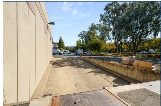
One of Two Exterior Dock Bays
