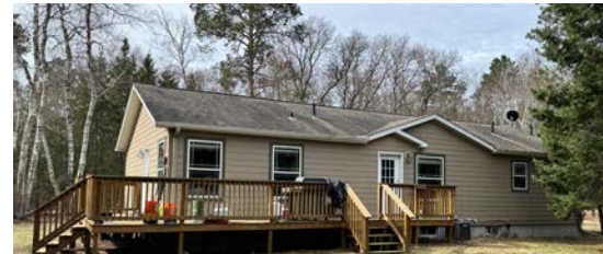
Ranger Residence and Office
