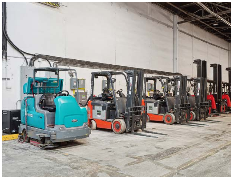
Zone 3: Charging station
