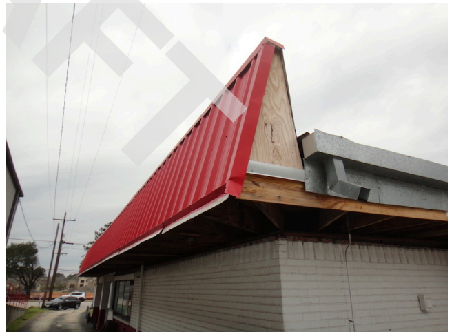
12. Roof parapet wall
