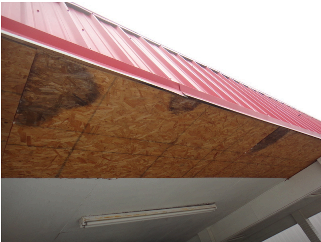
11. Damaged soffits
