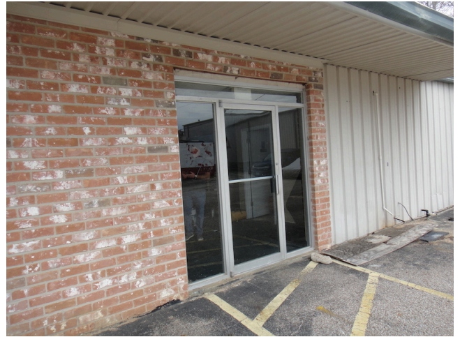
38. Entrance door and windows
