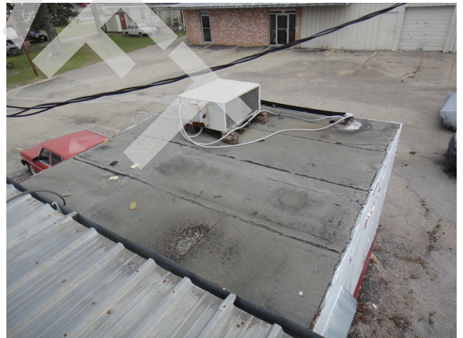
56. Walk in cooler roof
