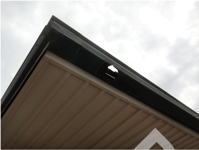
17. Damaged gutters
