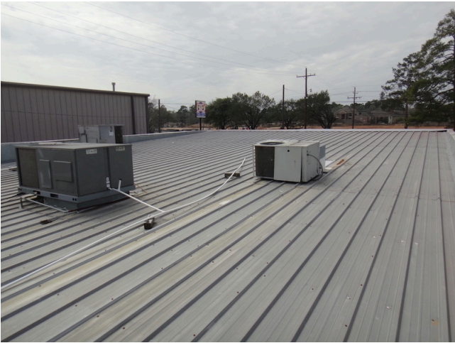
30. Corrugated metal roofing bldg 1
