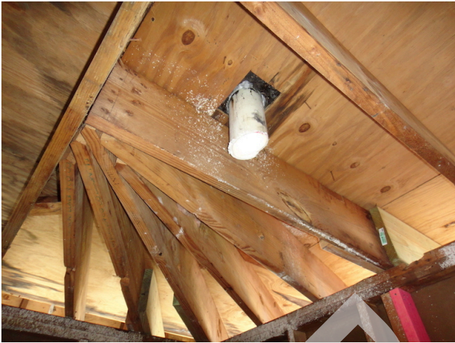
45. Plumbing removed bldg 1
