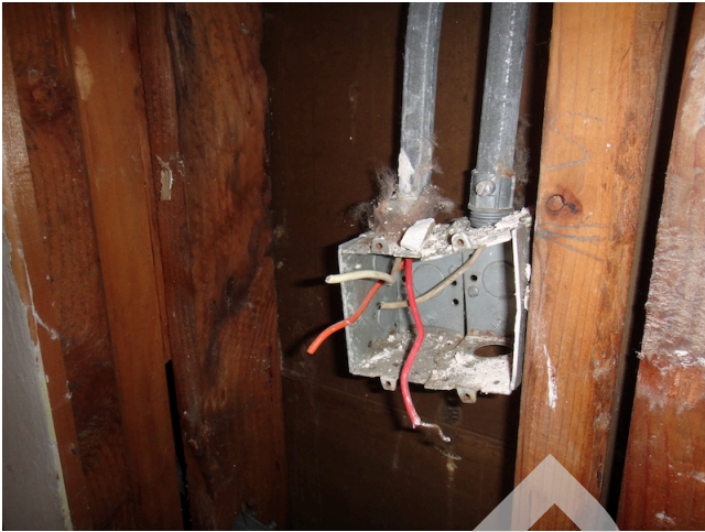
37. Electrical removed bldg 1
