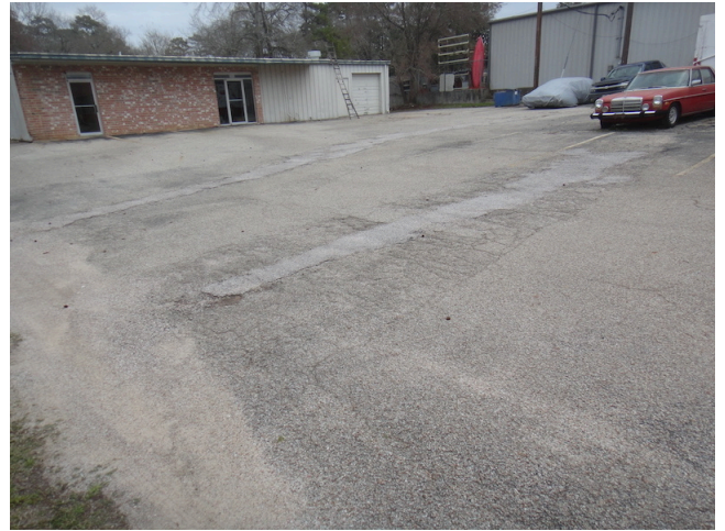
6. Fair asphalt paving
