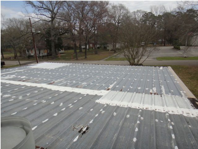
31. Corrugated metal roofing bldg 2
