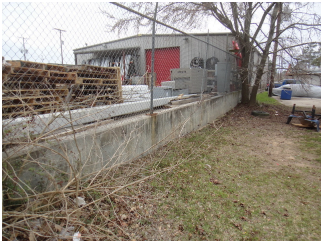
27. Concrete retaining wall along south
