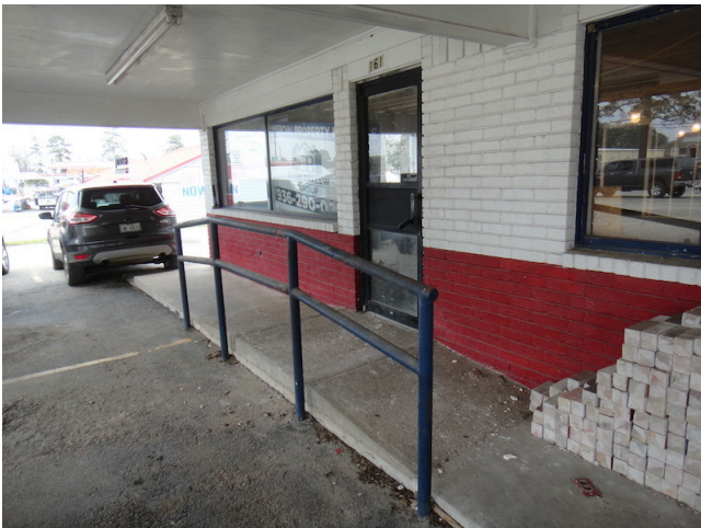
39. Entrance doors bldg 1
