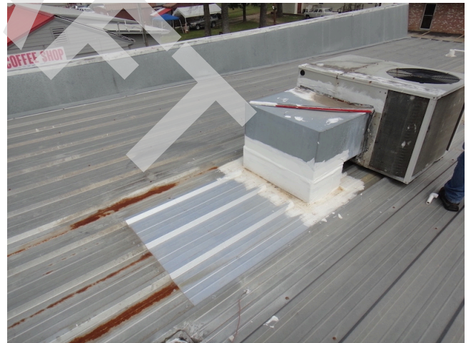
52. Roof repairs bldg 1
