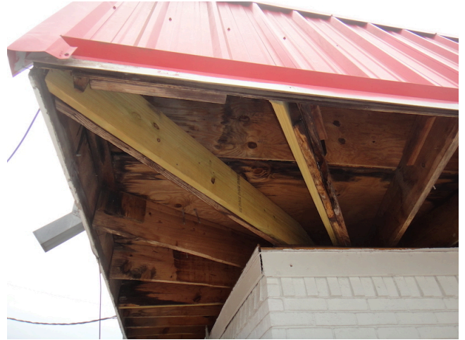
50. Recent framing repairs
