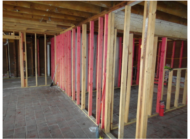
58. Wood framing bldg 1
