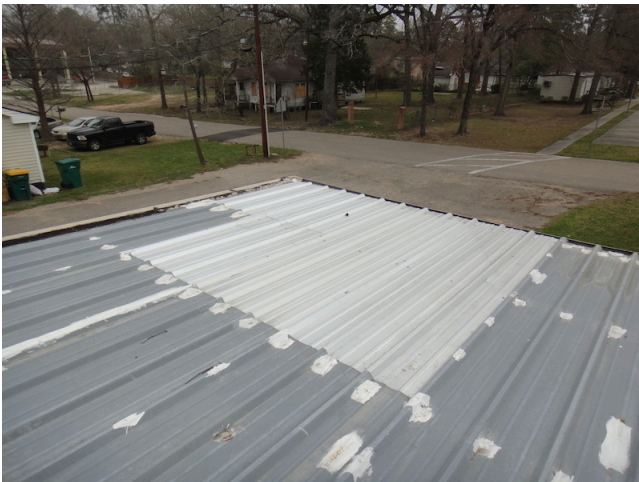
51. Recent roofing repairs bldg 2
