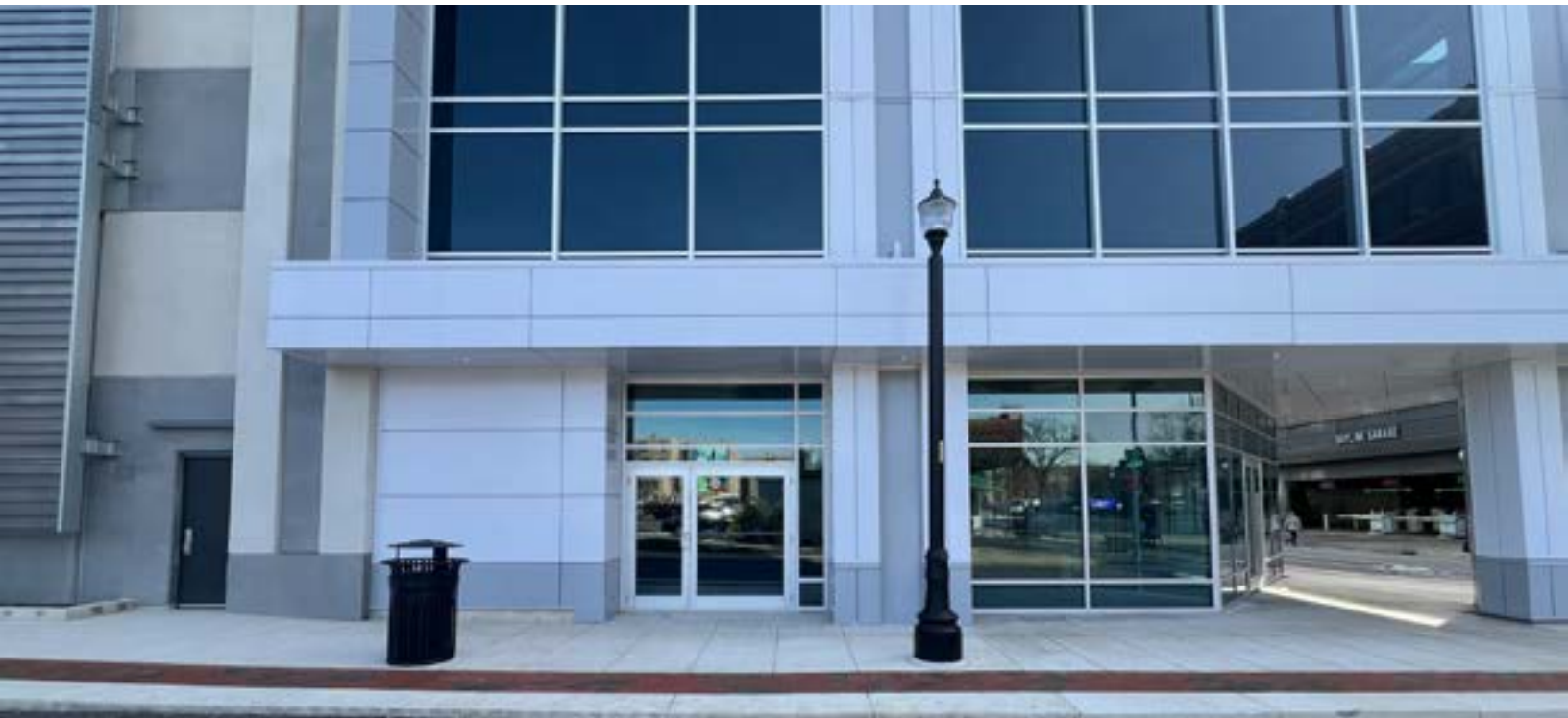
West Entrance - Maiden Lane showing dealer door
