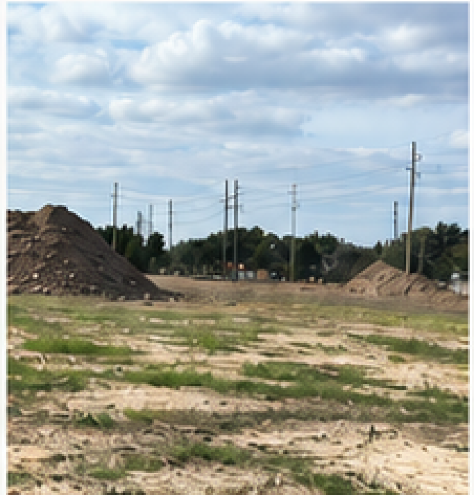
Site view – September 2026
