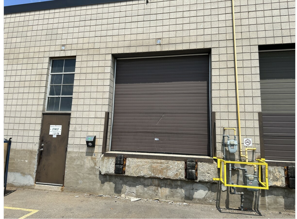
External Building Photo
