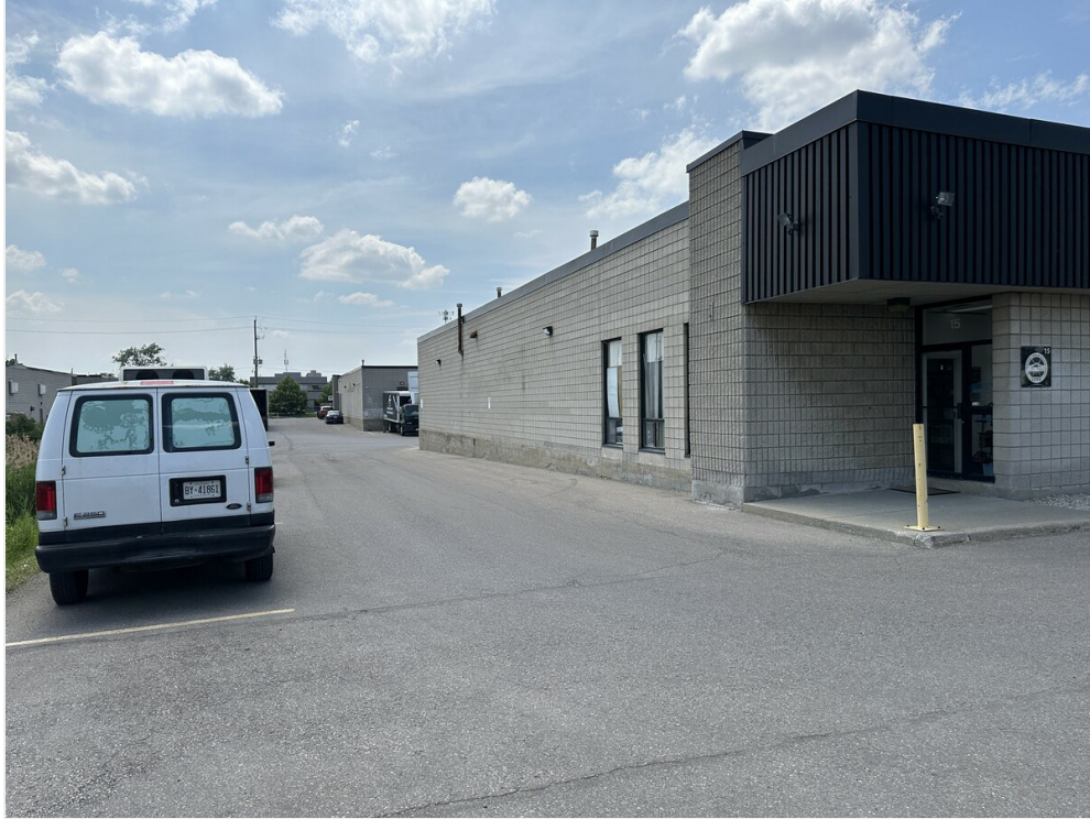
External Building Photo
