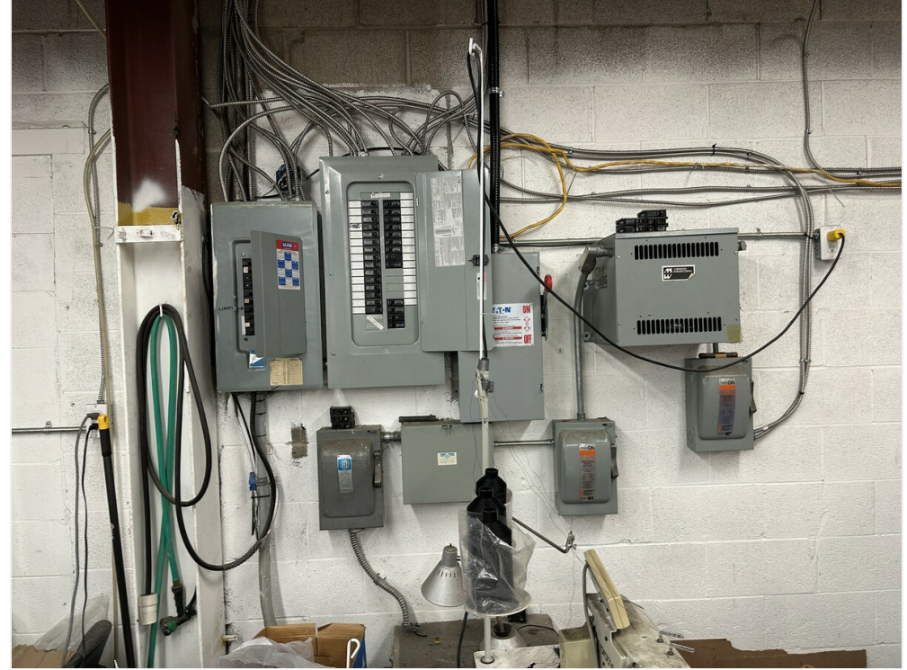
Internal building Photo
