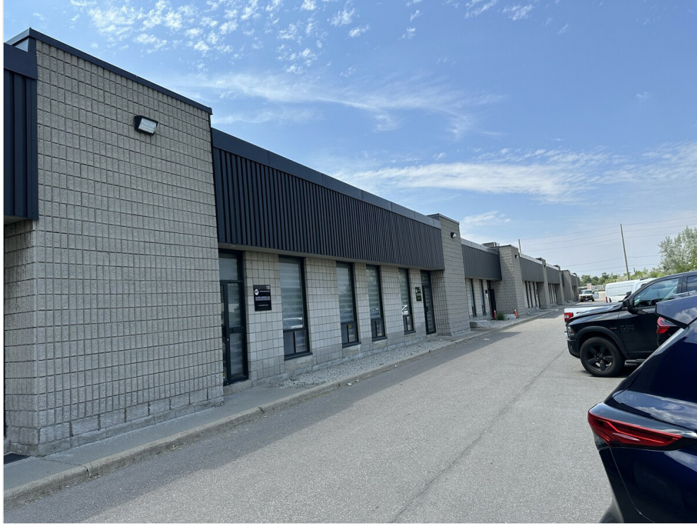
External Building Photo
