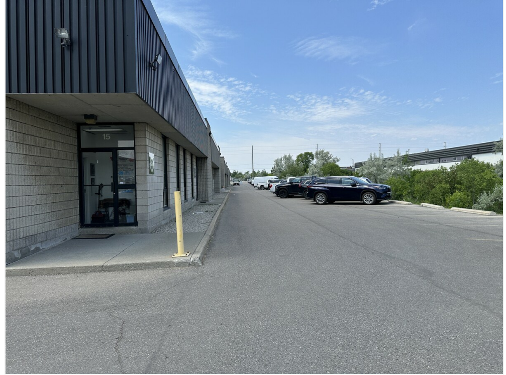
External Building Photo
