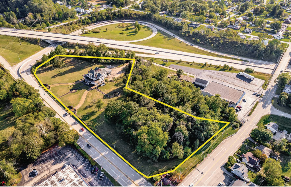
Aerial Facing South Towards Route 40.
