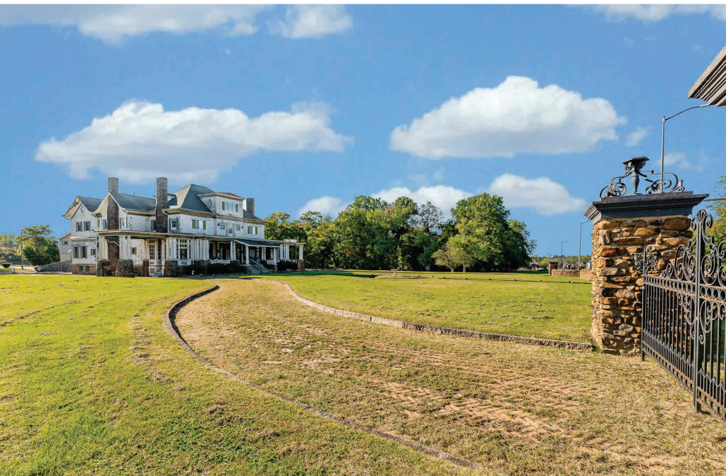
Exterior Front of the Building.
