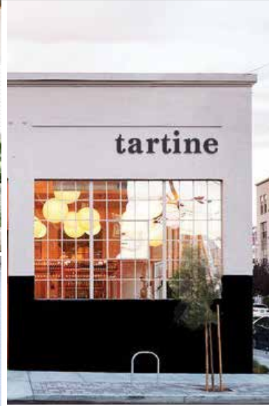
CREATING HEIGHT BY BUILDING A PARAPET WALL FOR MAIN SIGNAGE
