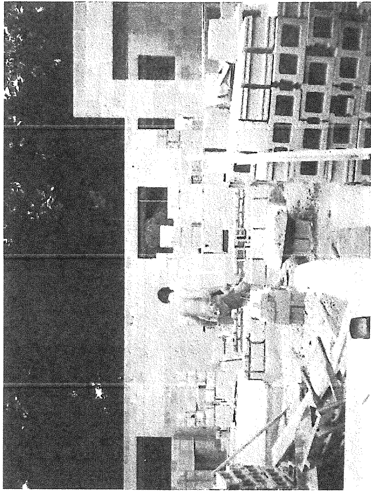
The building during construction shows the concrete block exterior walls.
