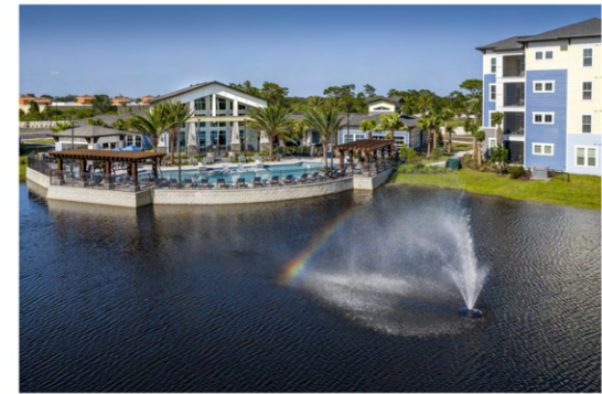
Integra Myst - .85 Mi 300 Apt. Units Under Construction
