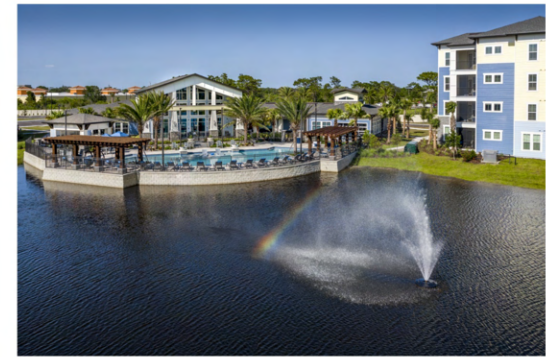
Integra Myst - .56 Mi 300 Apt. Units Under Construction
