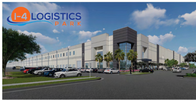
I-4 Logistics Park - .18 Mi Under Construction
