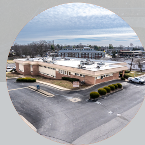
GROUND LEVEL ACCESS ALL SUITES
