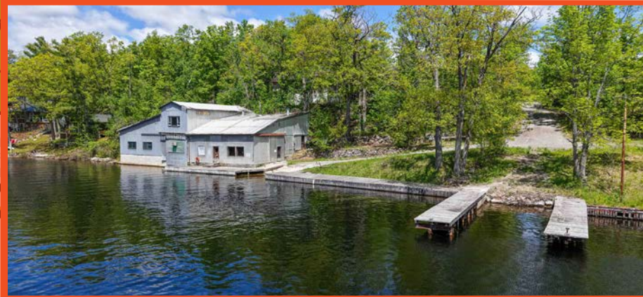
Former Marina 832 Northey's Bay Road
