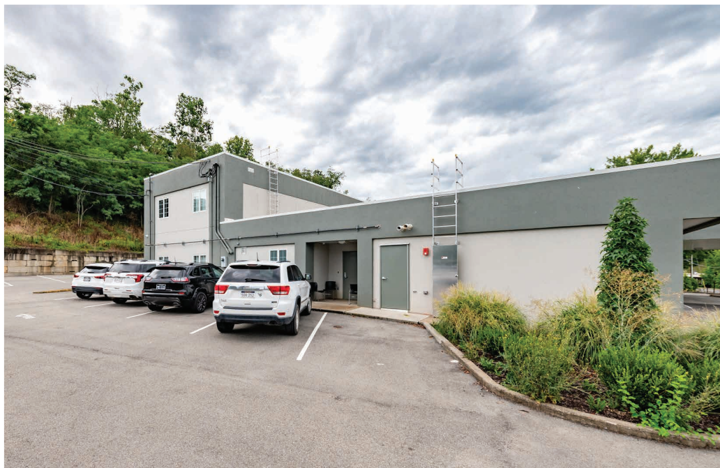
Side of the Building
