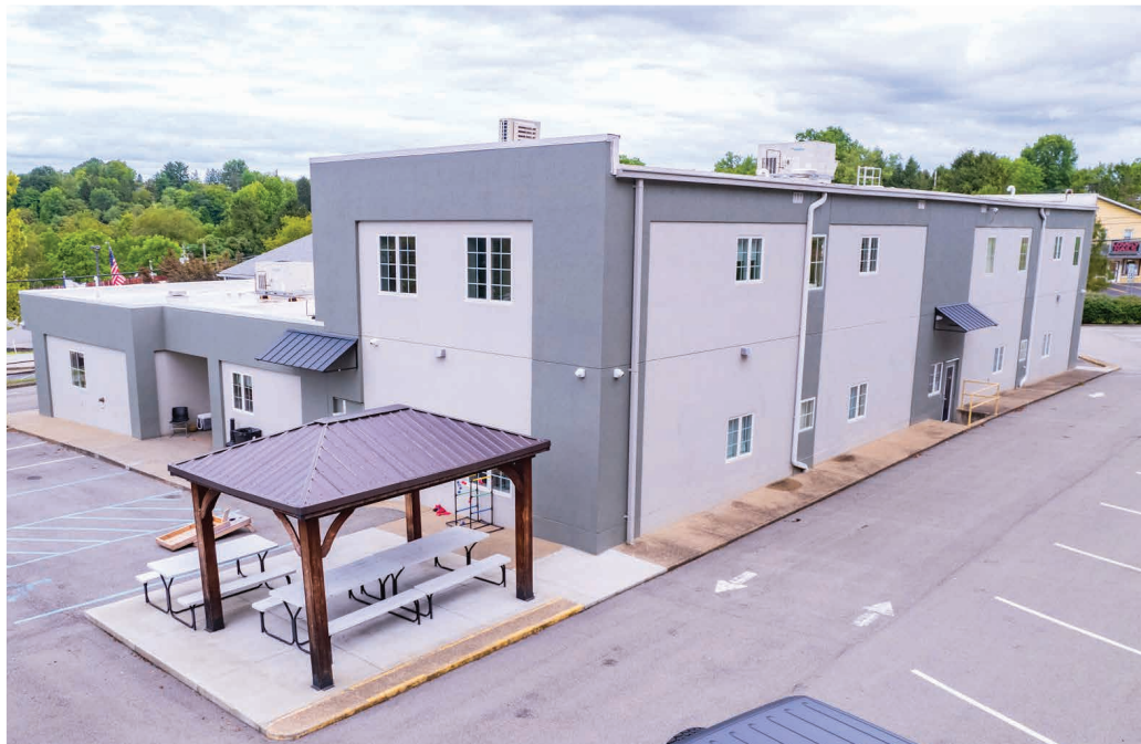
Back of the Building
