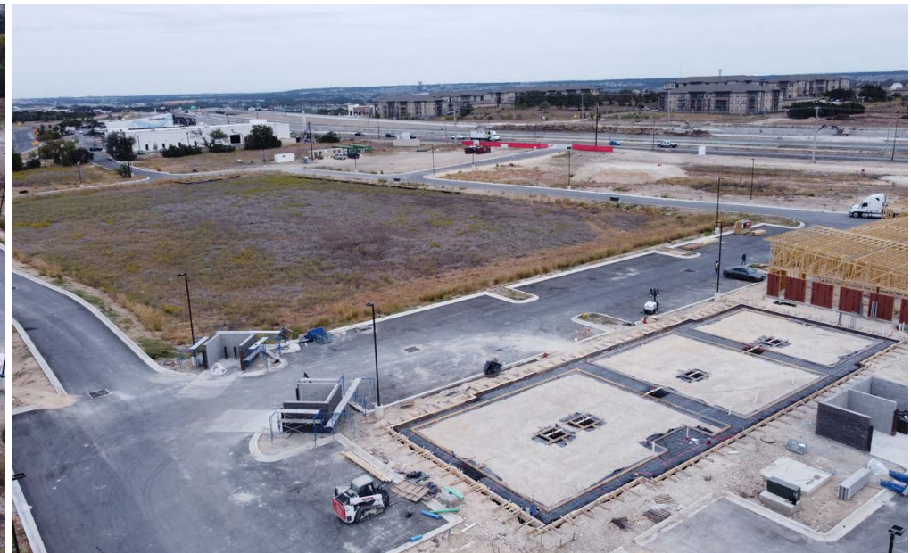
Construction Progress Oct 2024
