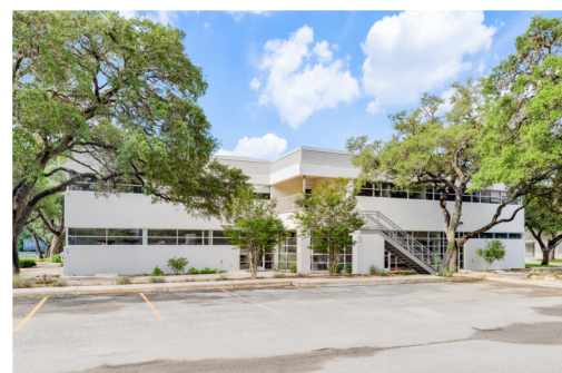
Two exterior entrances First and second floors
