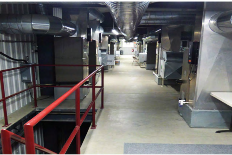
SECOND FLOOR MECHANICAL MEZZANINE
