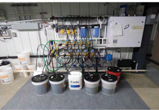
GROWLINK FERTIGATION SYSTEM
