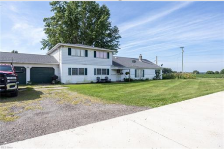
Front of Structure
