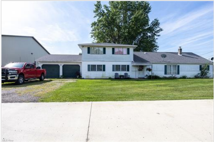
Front of Structure
