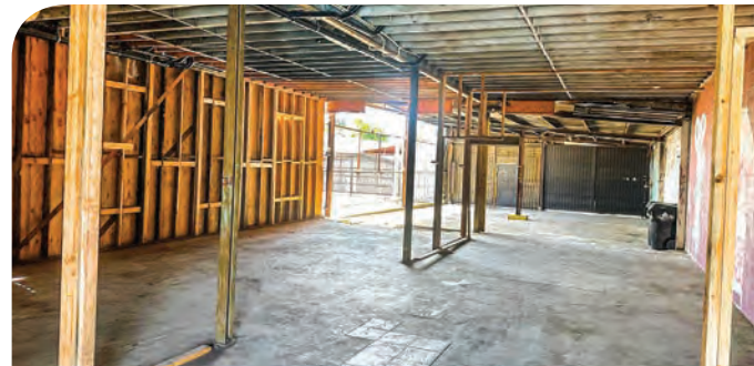
1424 W Slauson Ave - Interior View
