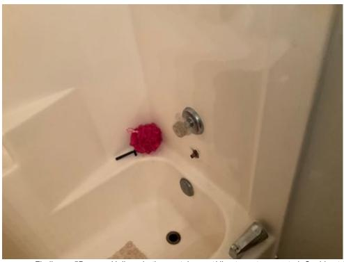
Finding: 5B Hallway bathroom tub spout/diverter not connected. Could not test shower head
