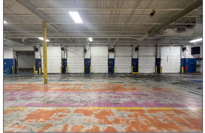
Main Warehouse Dock Area
