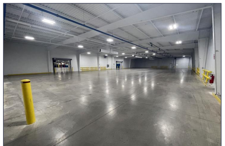
New Manufacturing Expansion Area (Northeast corner)
