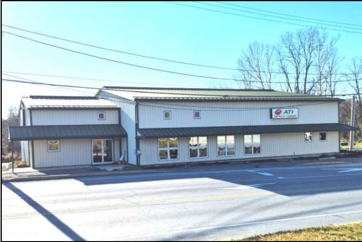
EAST SIDE OF 5,016 SQUARE FOOT BUILDING
