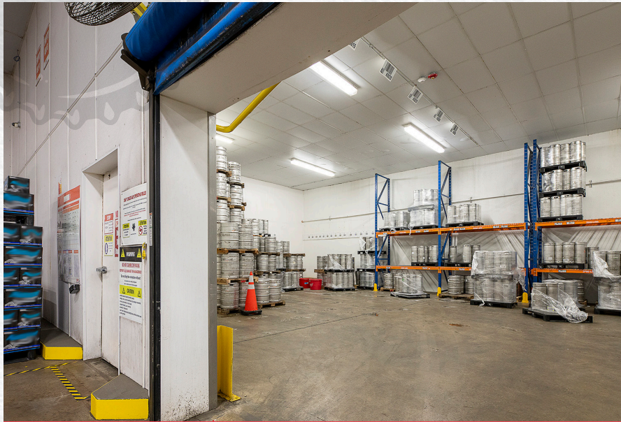
49'3" X 35" DRAFT COOLER ROOM - KEPT AT ROUGHLY 34 TO 36 DEGREES YEAR-ROUND
