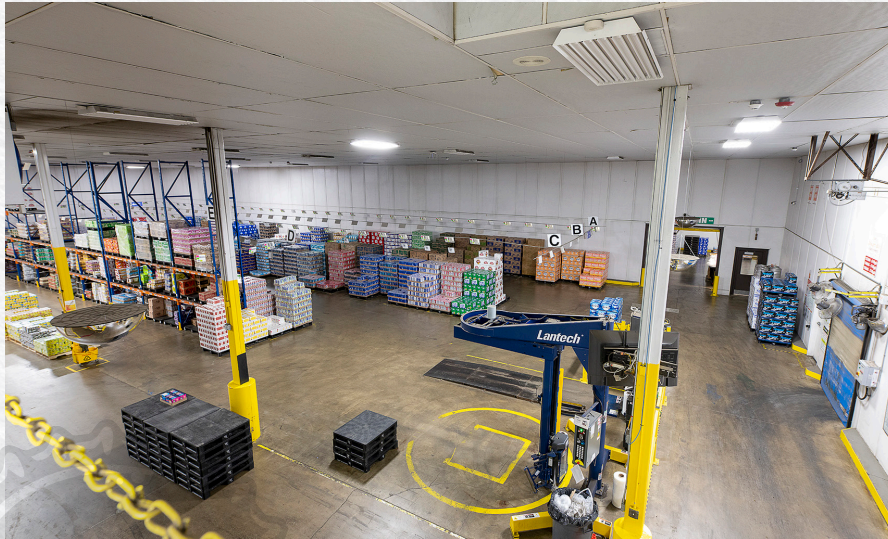
WAREHOUSE FEATURES LED LIGHTING
