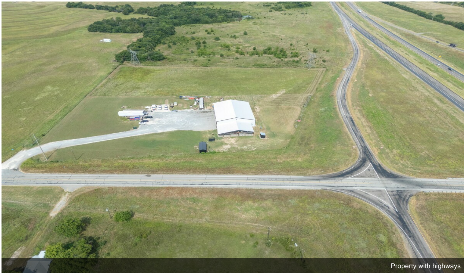
Property with highways
