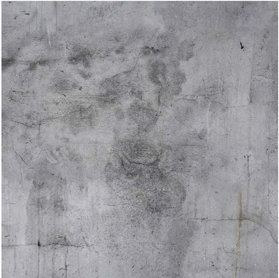
5 COLORED CONCRETE FLOOR EXPOSED CONCRETE CEILING
