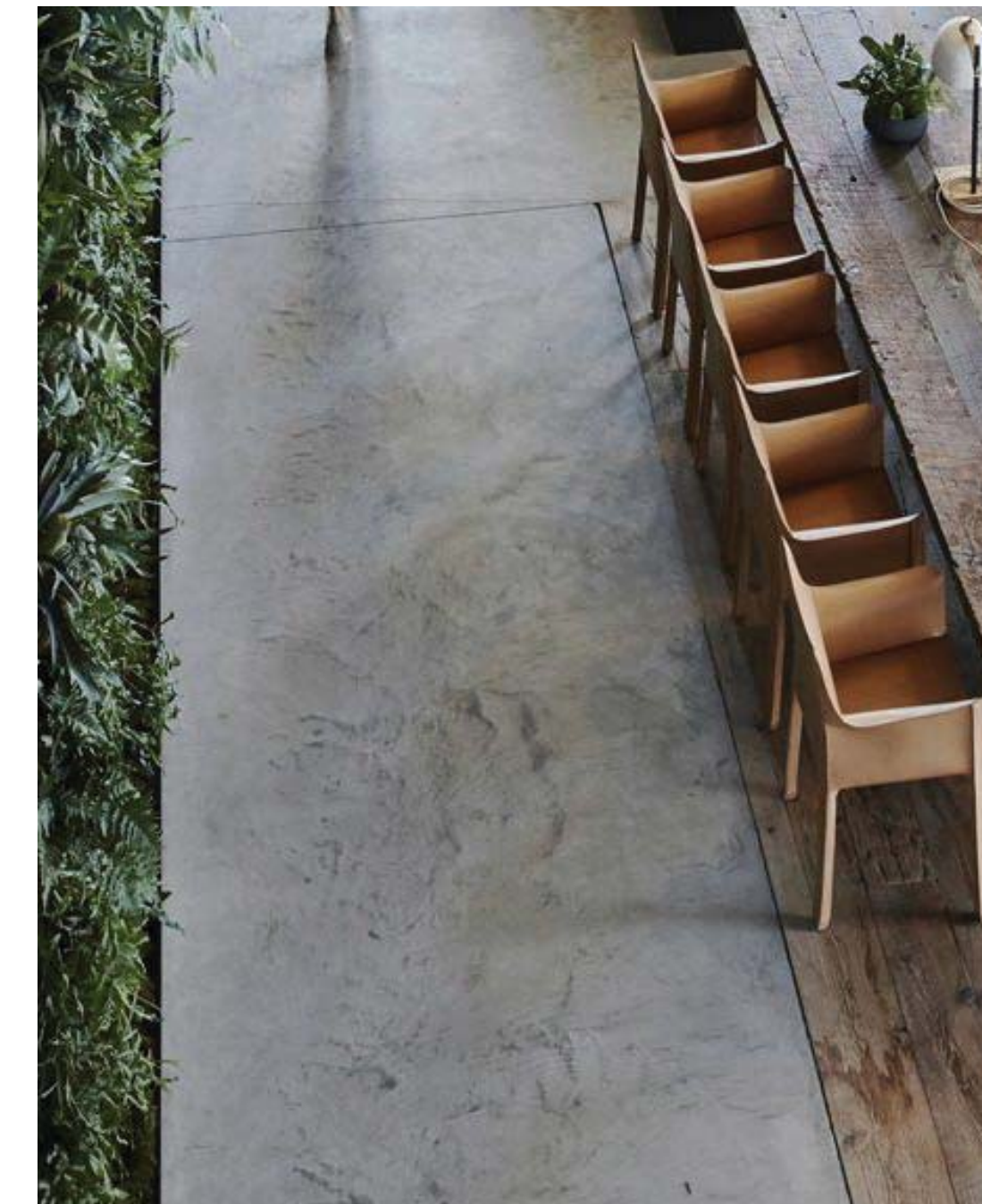
FLOOR: COLORED CONCRETE & RECESSED RECLAIMED WOOD
