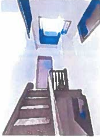
Other - Staircase to 4th floor with skylight to rooftop.
