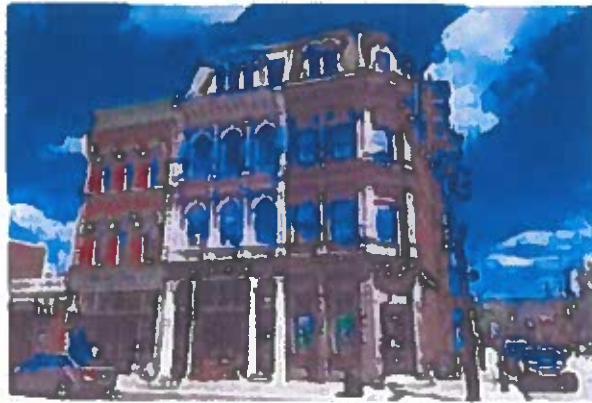
Front of Structure - The 1st floor tenant is a thriving coffee/cafe shop also occupying the mezzanine 1/2 floor.
