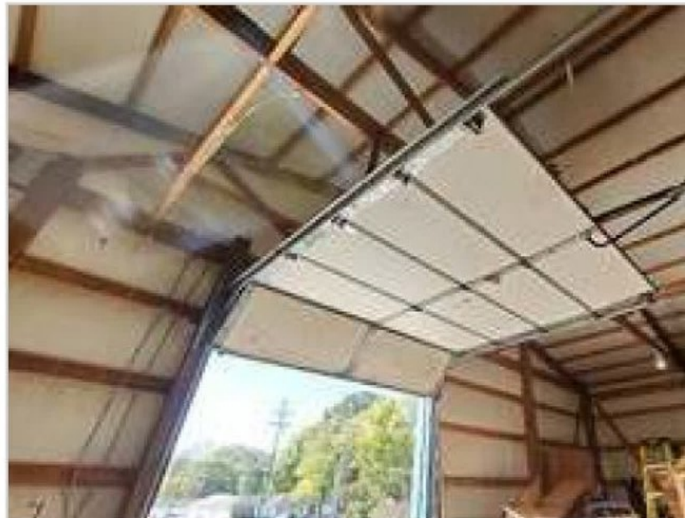
Storage building overhead door
