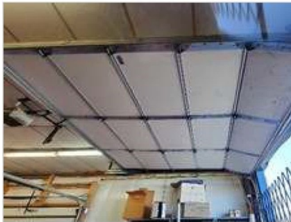
Rear side overhead door
