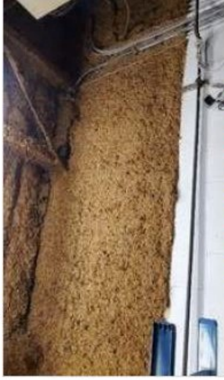
Front stockroom, spray-on insulation
